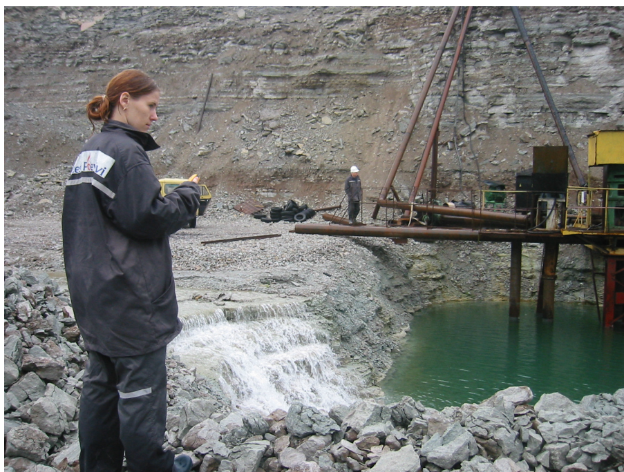
Fig. 3. Pumping station of Aidu open cast, area observation and field measurements (picture taken by Mining department of Tallinn University of Technology).
