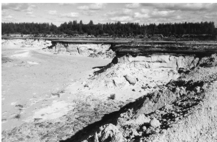
Fig. 3. Technogenic valley formed after sand flow into the trench in March 1999
