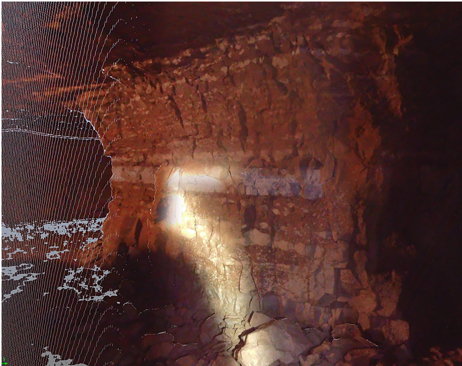
Fig. 10. A high-resolution TLS point cloud of a pillar, the limestone interbed can be identified by a centrally (at the height of 1.6 m from the mine floor) located bright layer.
